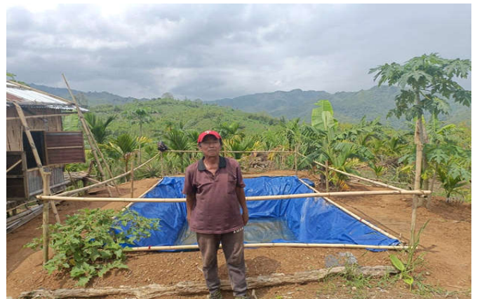
Dug out pond for rainwater harvesting
