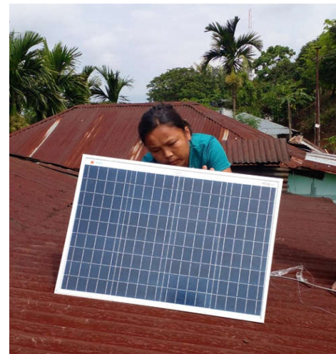
Home Lightning System Instillation by Sakawrdai Solar Mama
