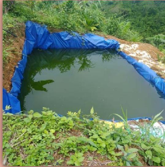
*FIG: Dug out pond for rain water harvesting is introduced in the project area as most crops are rain fed.*
